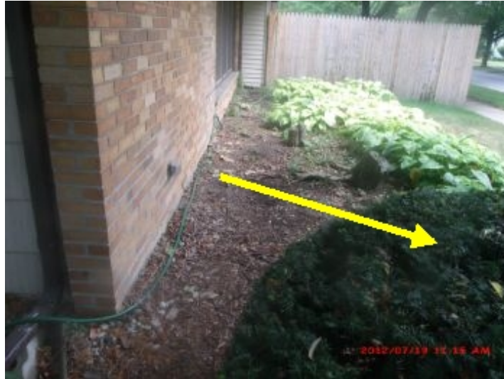
right (east) side graded generally away from foundation
