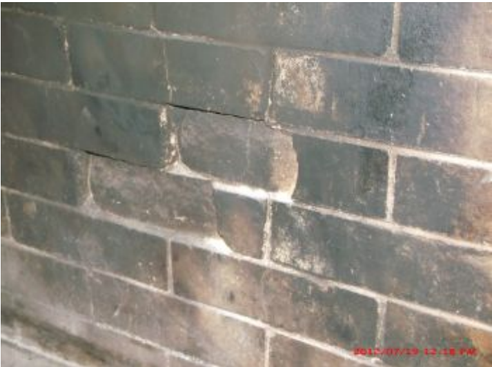
Some Fireplace brick deterioration
