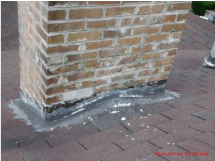
Flashing wear near chimney - suggest year maintenance
