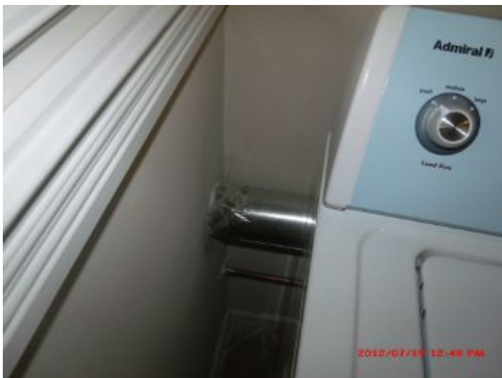
Dryer vent ductwork
