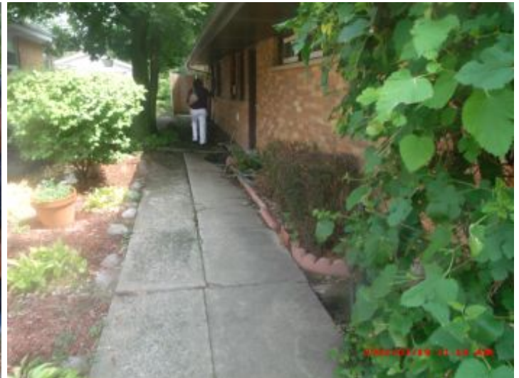
Left (west) side sidewalk graded towards house
