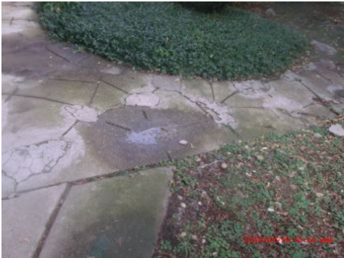
Concrete walkway cracks and patches
