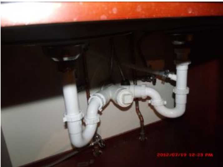
PCV waste pipe under sink
