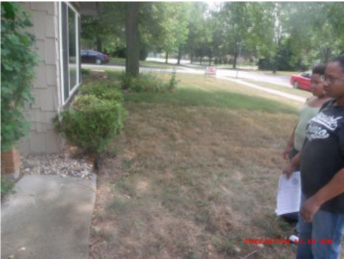
Front graded generally away from foundation
