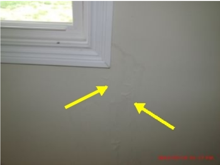
Signs of moisture leak - rear bedroom window
