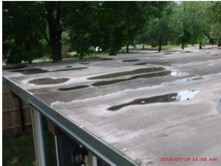
some water pooling on flat top
