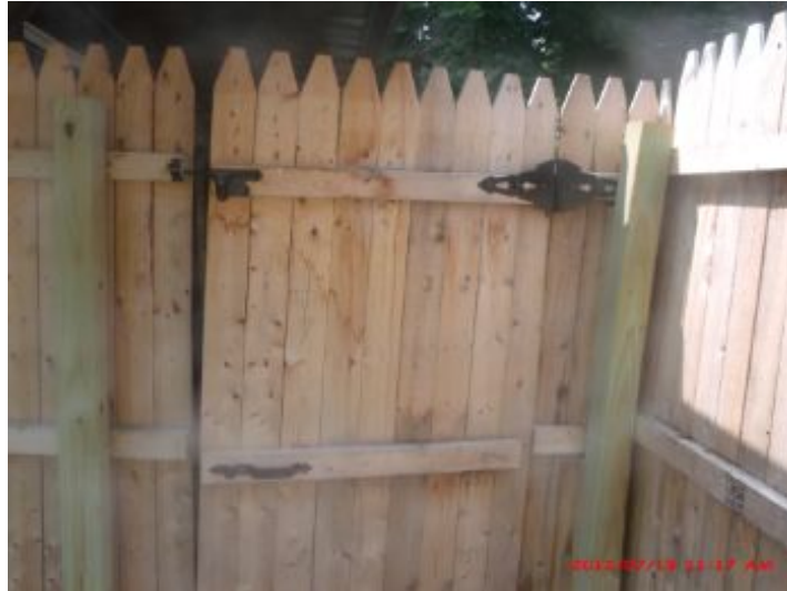
Gate out of alignment
