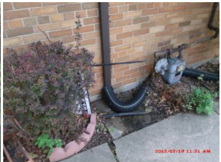
Extended downspout at front left (southwest)
