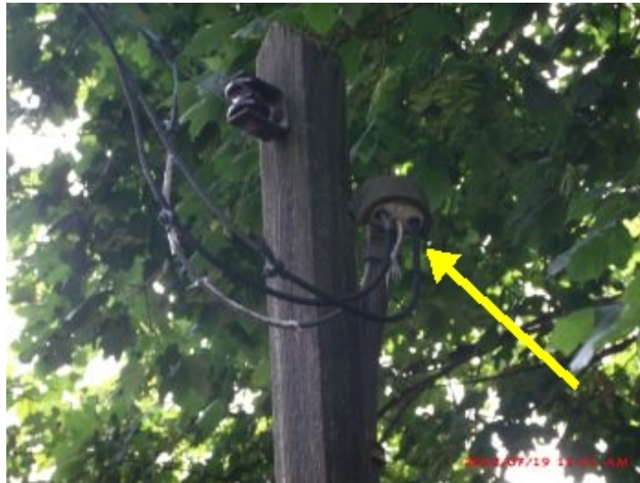
Overhead mast three wire (240 volt) system
