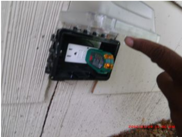
Testing exterior outlets
