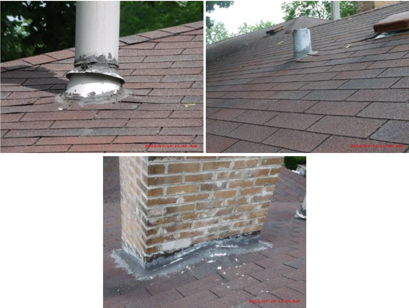
Flashing wear near chimney - suggest year maintenance
