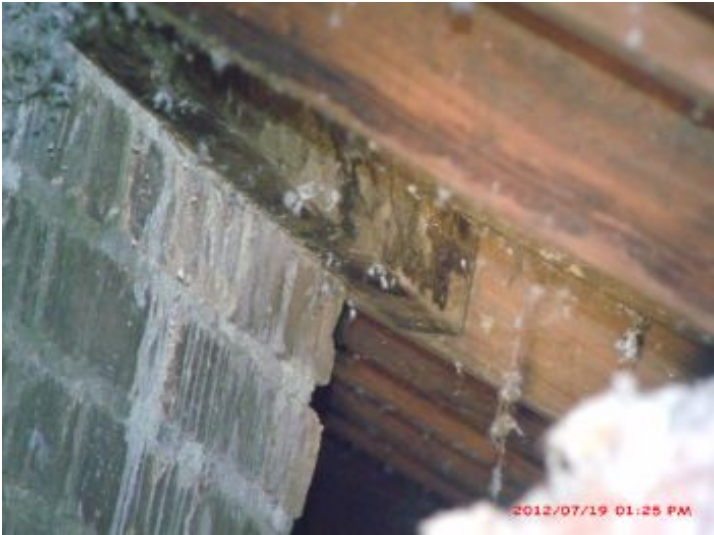
Evidence of past leaking
