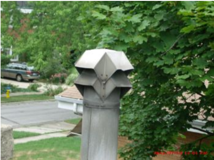
Furnace chimney cap
