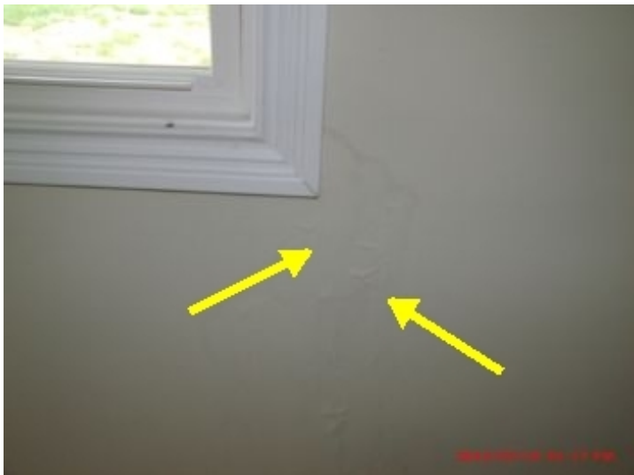
Signs of moisture leak - rear bedroom window
