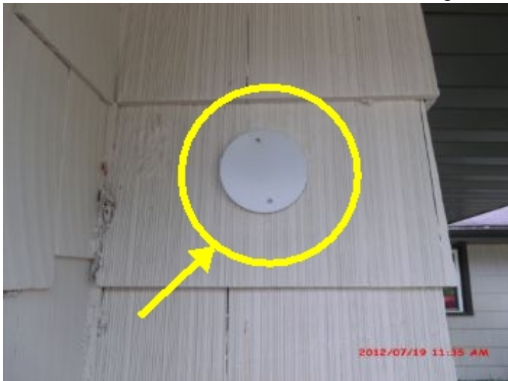
Suggest sealing patches to prevent moisture intrusion
