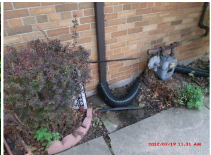
Extended downspout at front left (southwest)
