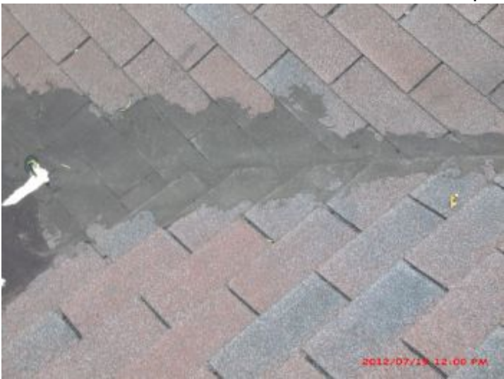
Some indication of repair in valley near flat top
