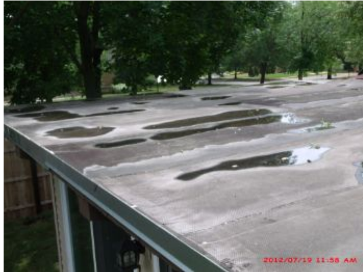
some water pooling on flat top
