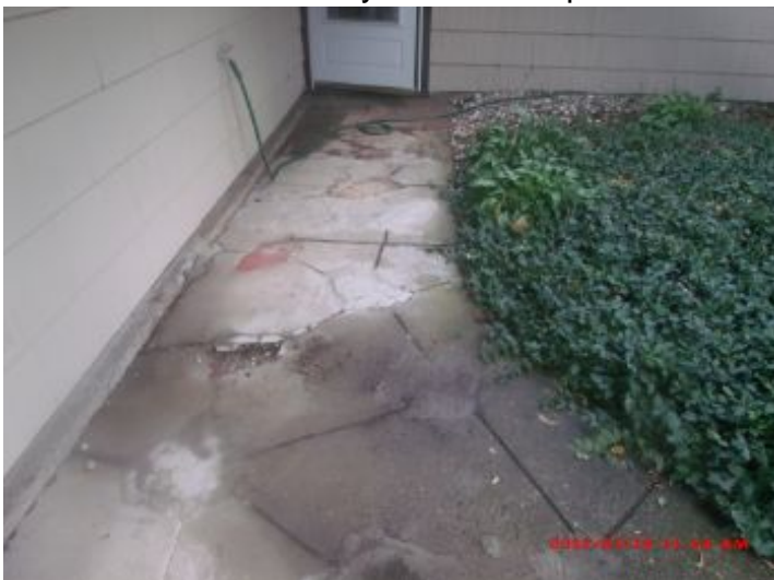
Concrete walkway cracks and patches
