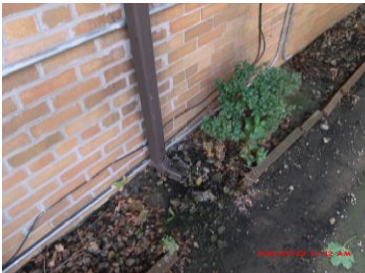
Suggest extending downspout to deposit water away from building
