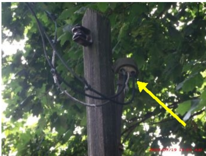
Overhead mast three wire (240 volt) system
