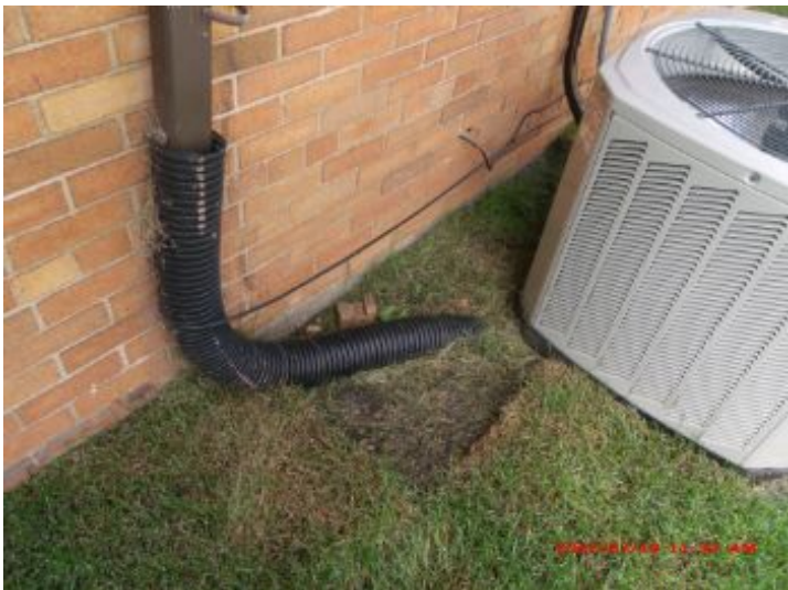
Downspout in rear appears to be blocked. Suggest opening up to deposit away from building
