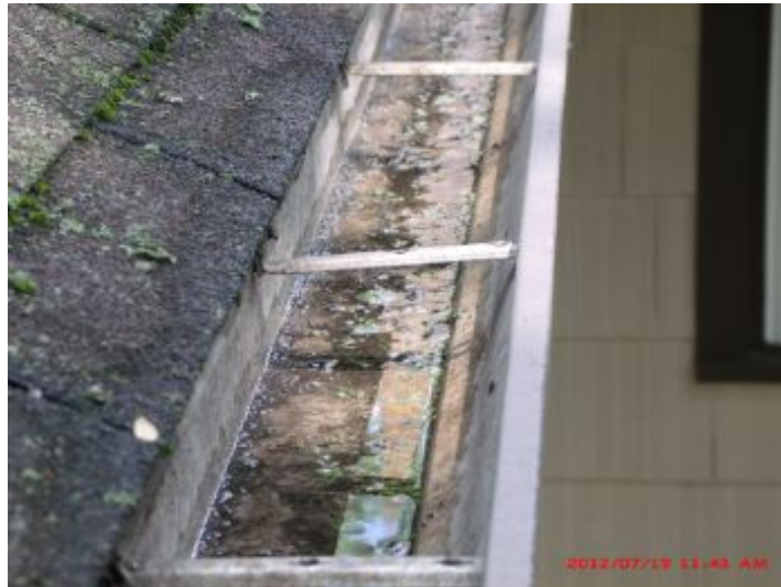
Some asphalt sand in gutter, indicative of recent roofing
